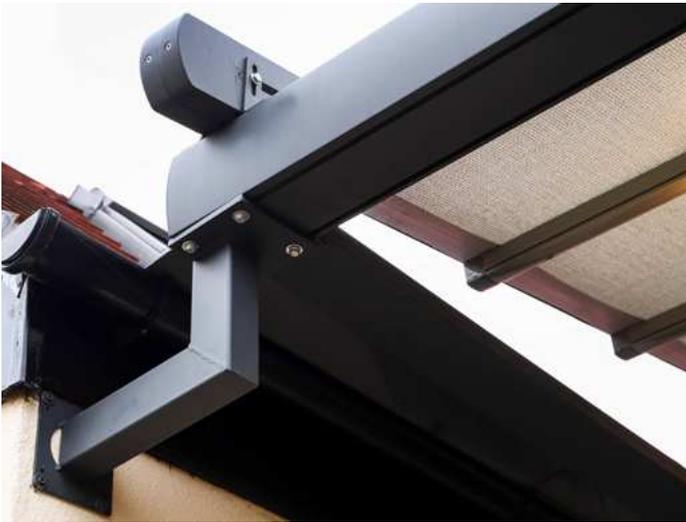
In this project, the front post of the left side pergola has been removed and replaced with the L bracket attached to the wall. Middle post moved to the left 500 mm to avoid blocking glazing. Waterproofing provided by the L-shape panel between the wall and the pergola. (required due to WaterPipe)
